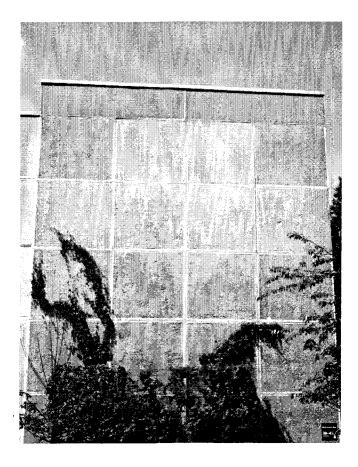
Fig. 4. Exterior grid of concrete panel construction.
